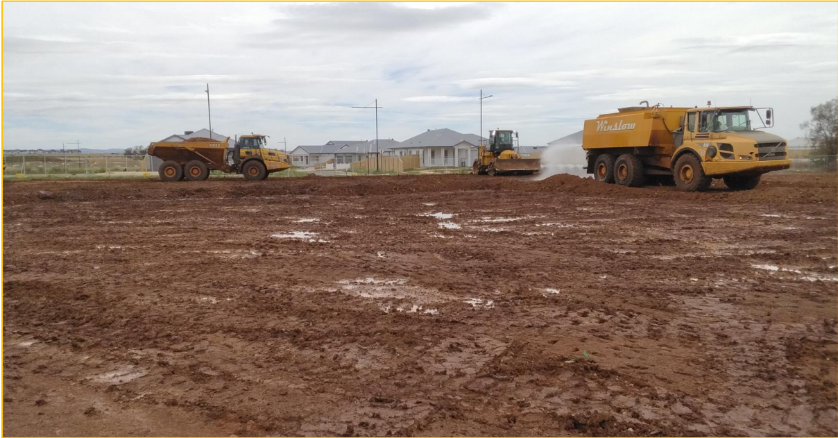
Figure 4: Fill Spreading & Moisture Conditioning (Source: CTGM)
