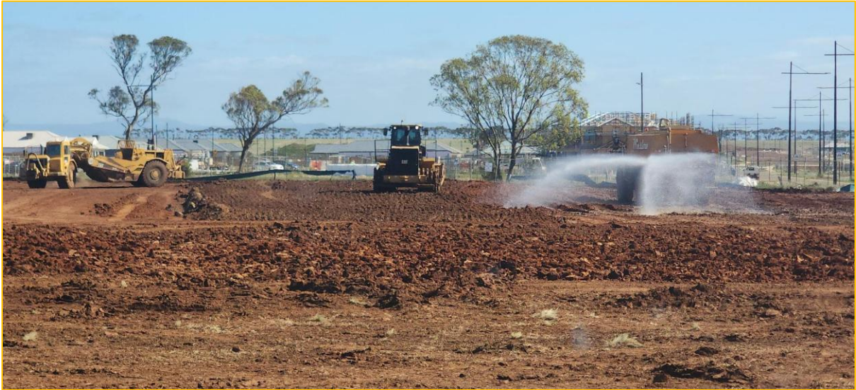
Figure 2: Filling Process Showing Compaction & Moisture Conditioning During Spreading (Source: CTGM)
