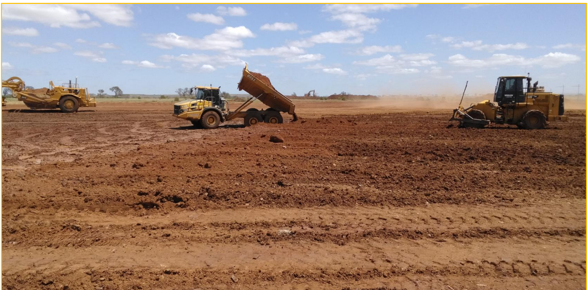
Figure 3: Fill Being Transported to Placement Zone (Source: CTGM)
