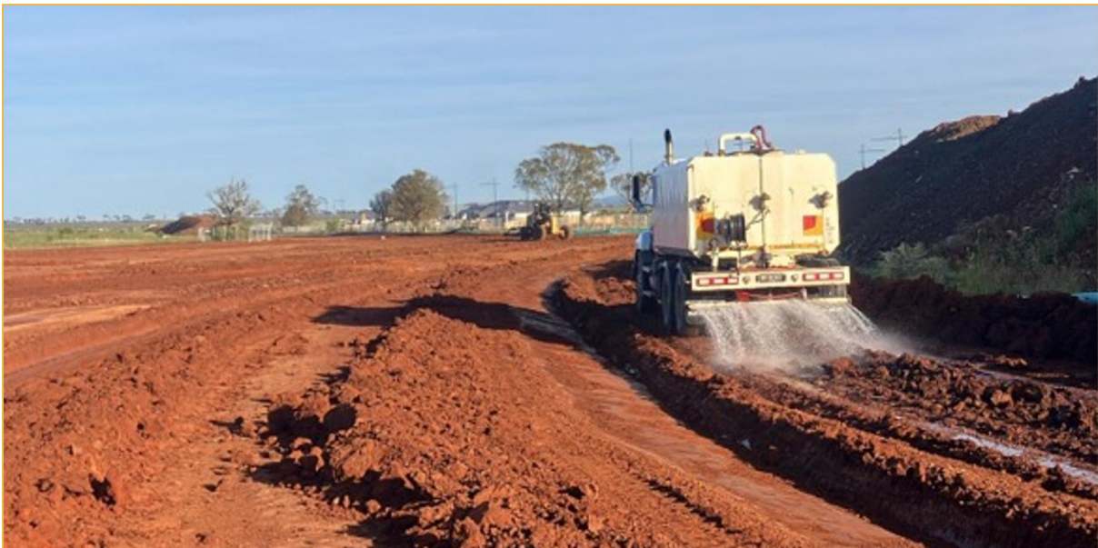
Figure 1: Moisture Conditioning of Subgrade (Source: CTGM)
